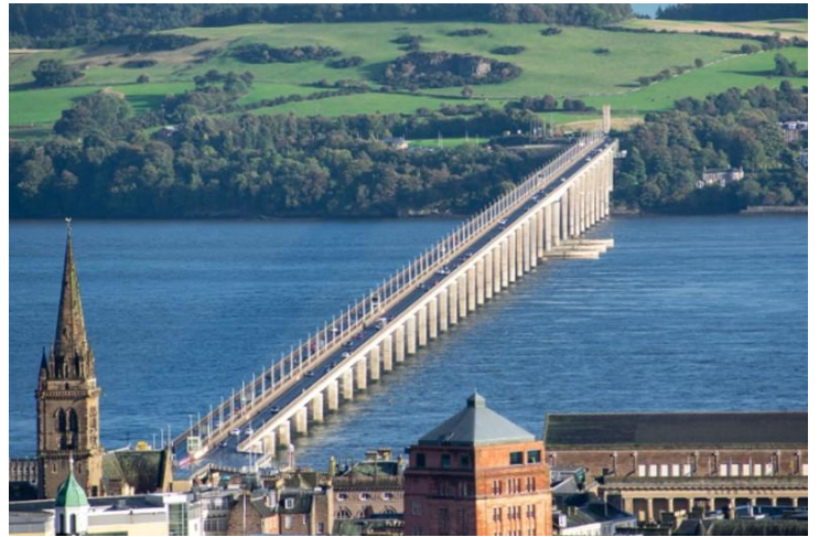
Tay Road Bridge at Dundee
