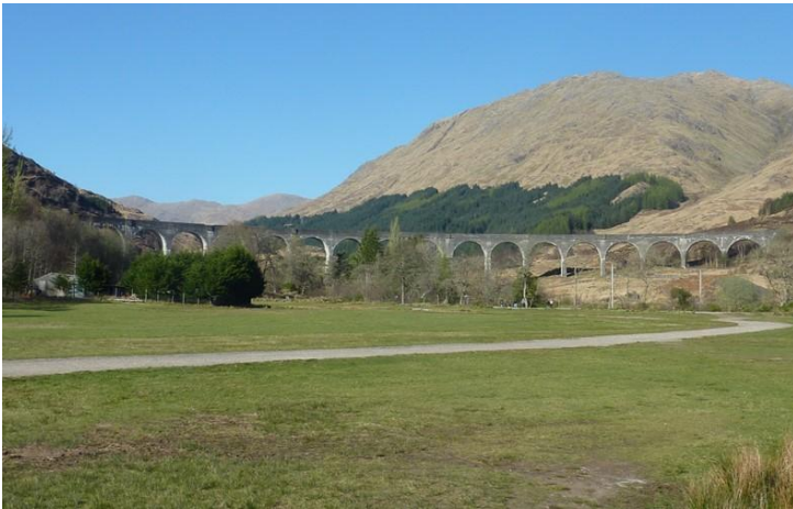
Glenfinnan Rail Viaduct
